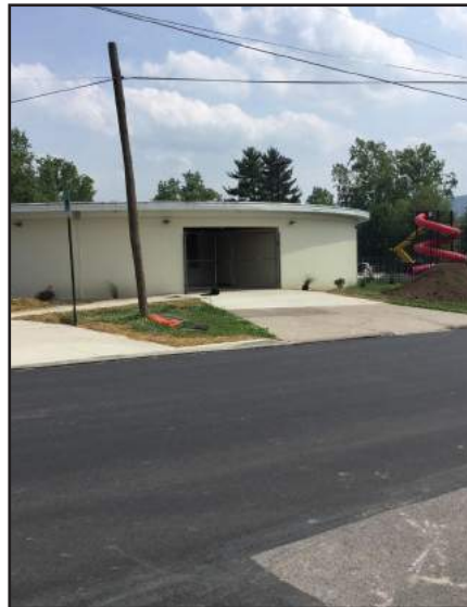
1700 W 4th Street 70-013-302 Pool House
