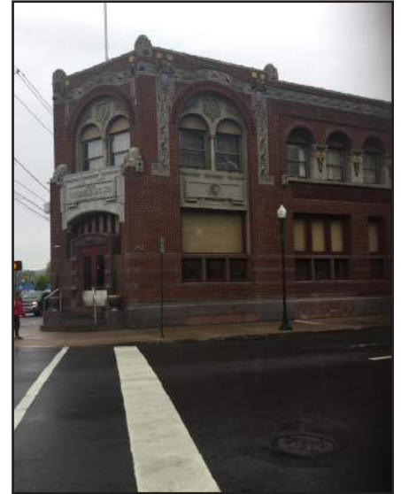
252 W 4th Street 63-007-402 Williamsport Sun-Gazette Building
