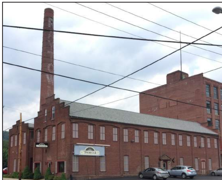
Photograph 6: The Pajama Factory building complex, formerly the Lycoming Rubber Company.
