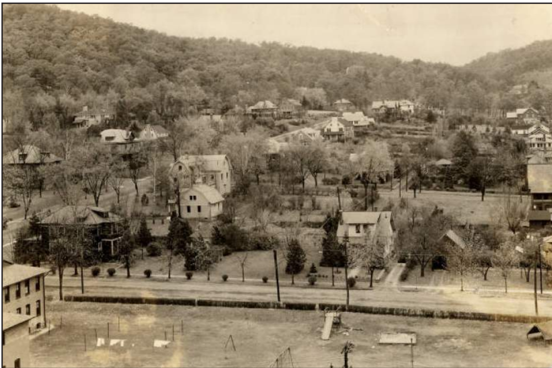
Photograph 1: 1933 bird's-eye view of the Vallamont neighborhood. (Source: James V. Brown Library)
