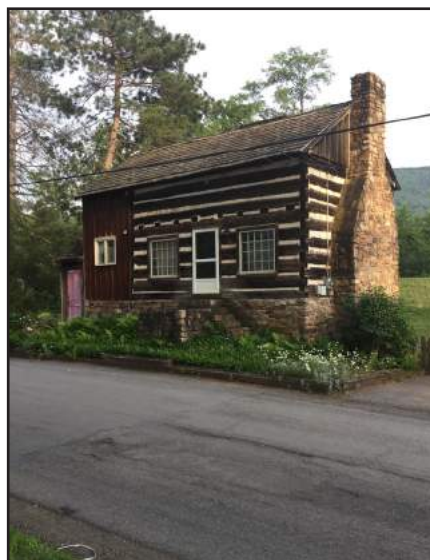
2886 S Reach Road 71-009-707 Log Granary of Old Mill
