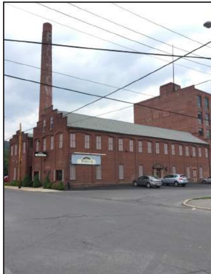
1307 Park Avenue 70-002-511 SHPO Eligible, 2009 - Key#035741
