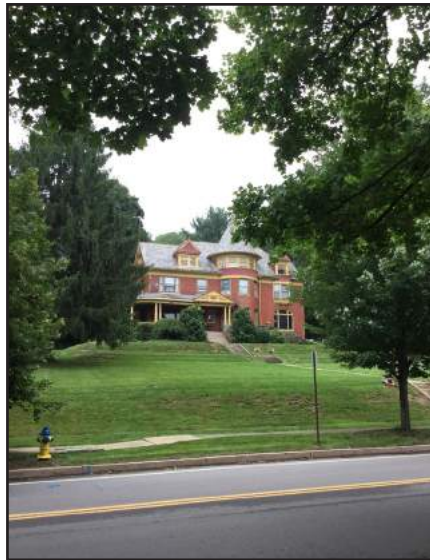
125 Grampian Boulevard 75-007-105 Schleh House
