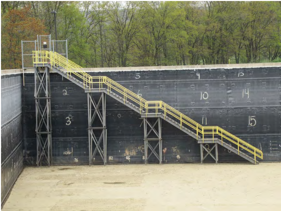
Western Stair Tower (Inside of Tank Looking West)
