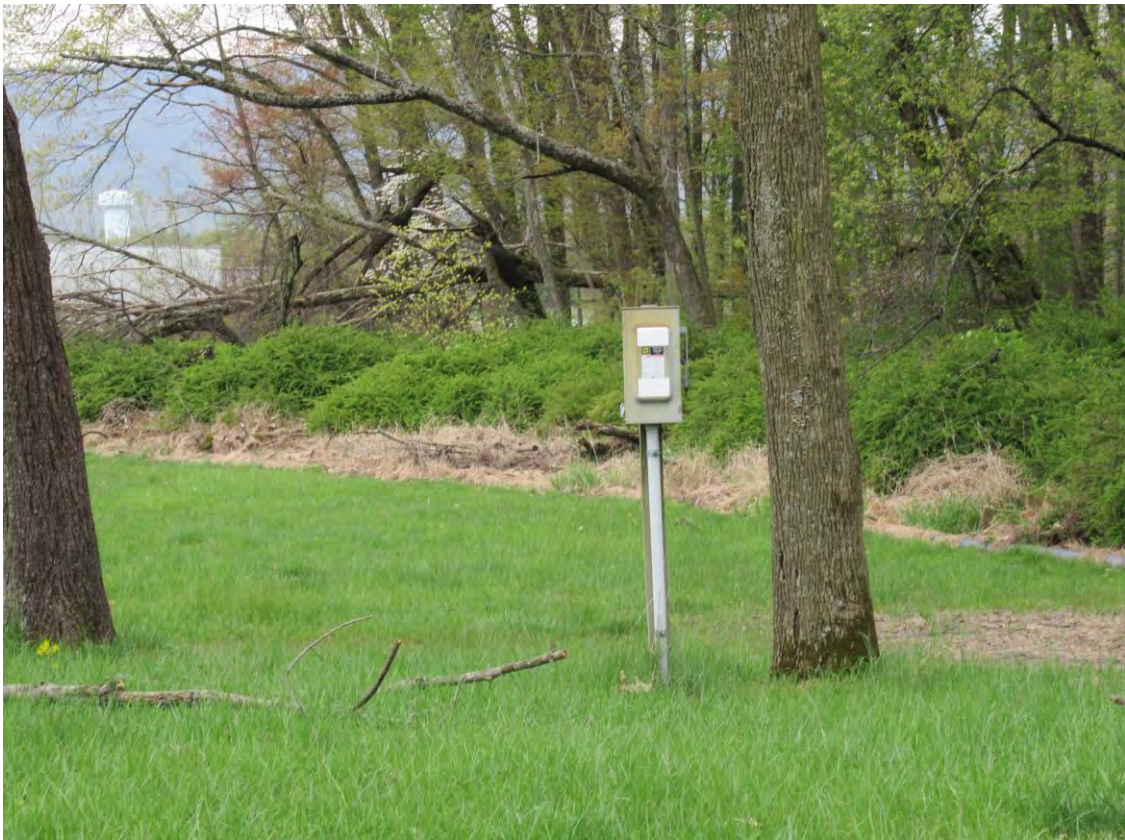
Electrical Disconnect for Contractors use
