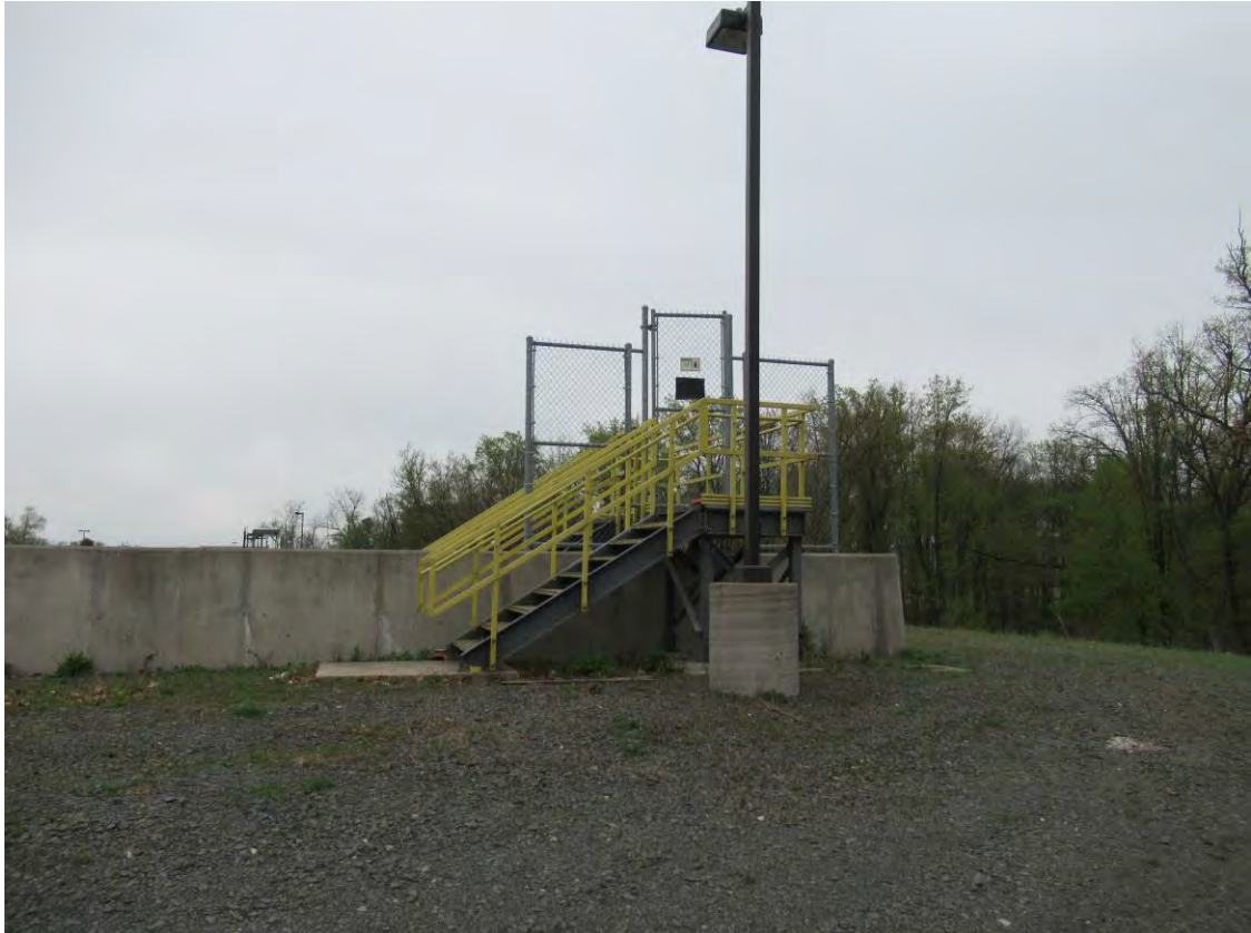
Western Stair Tower (Outside of Tank Looking East)
