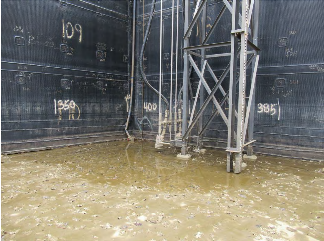
Sump Area (South East Corner)
