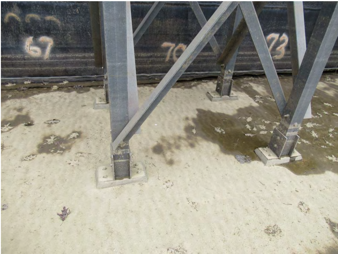
Stair Tower Legs
