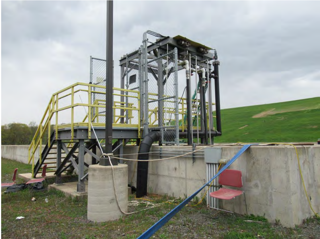
Eastern Stair Tower (Outside of Tank Looking North)
