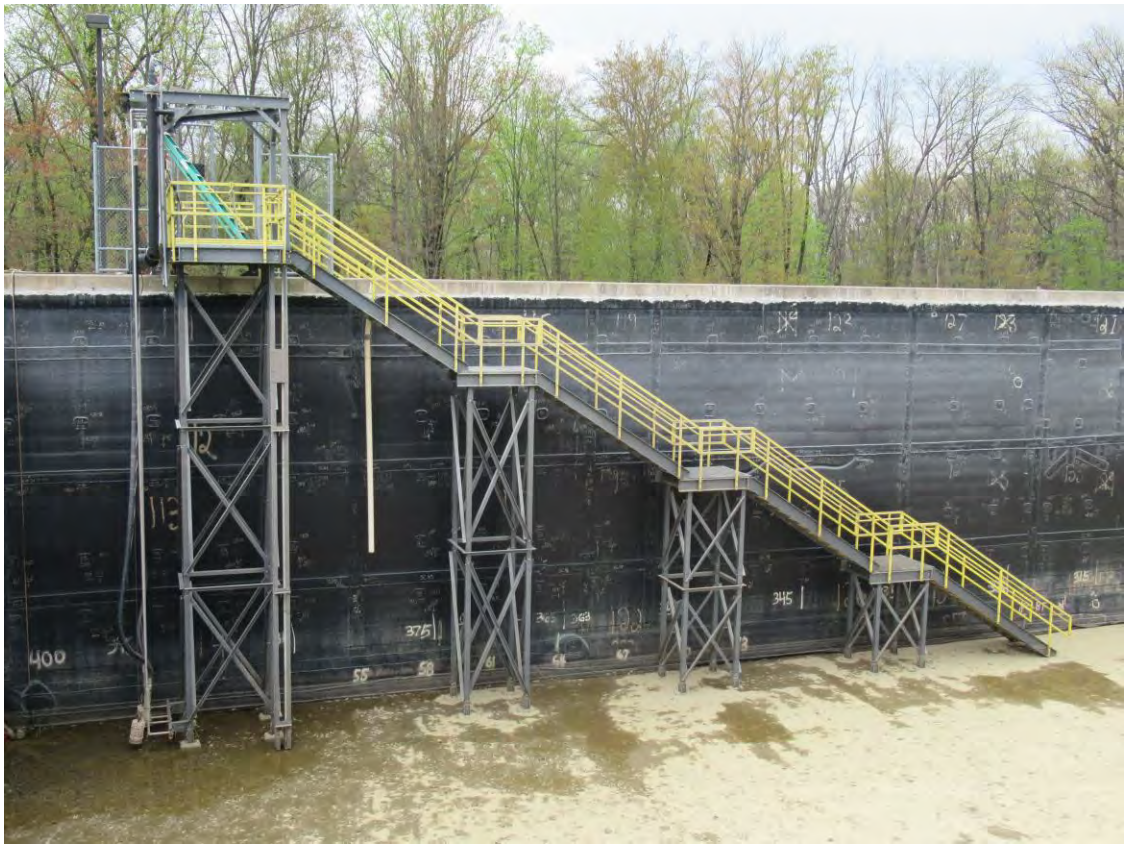
Eastern Stair Towers (Inside of Tank Looking South)
