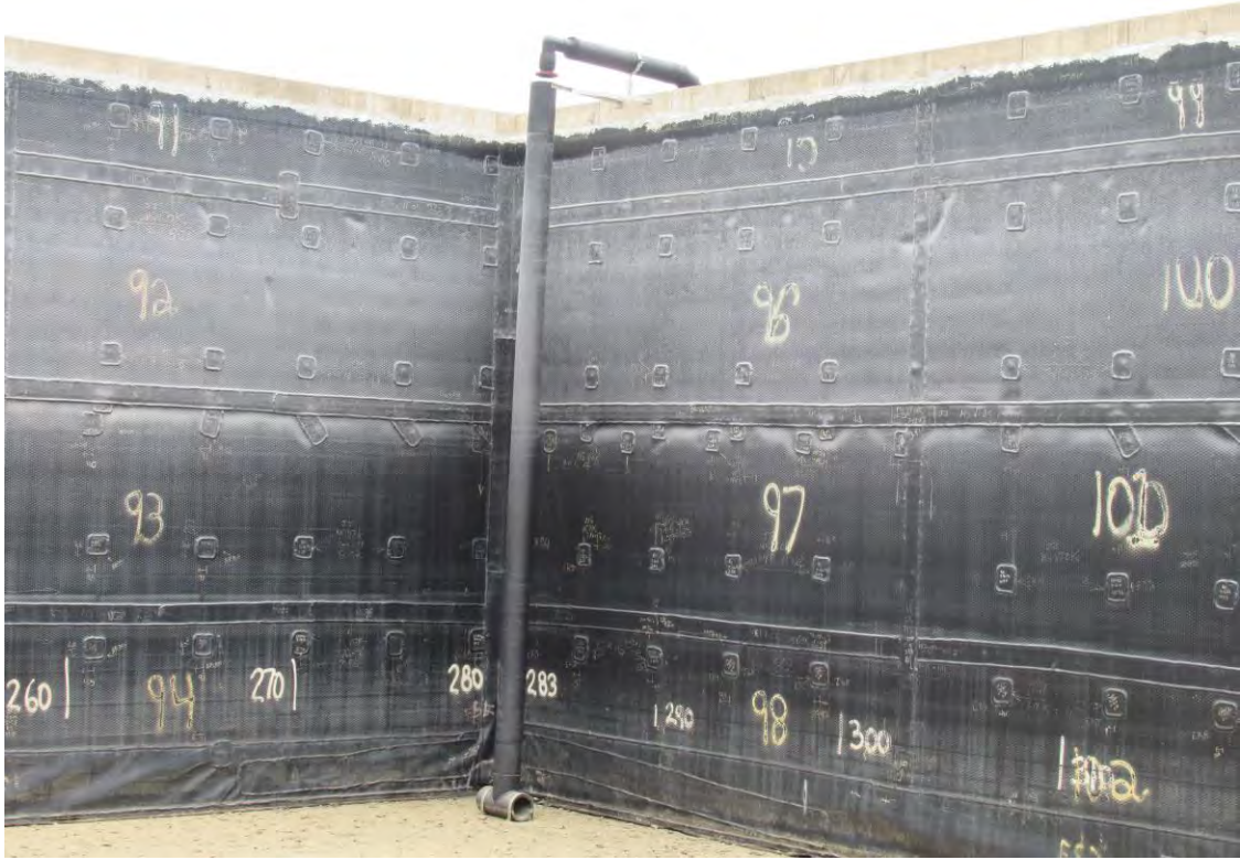
Permanent Fill Pipe (North East Corner)
