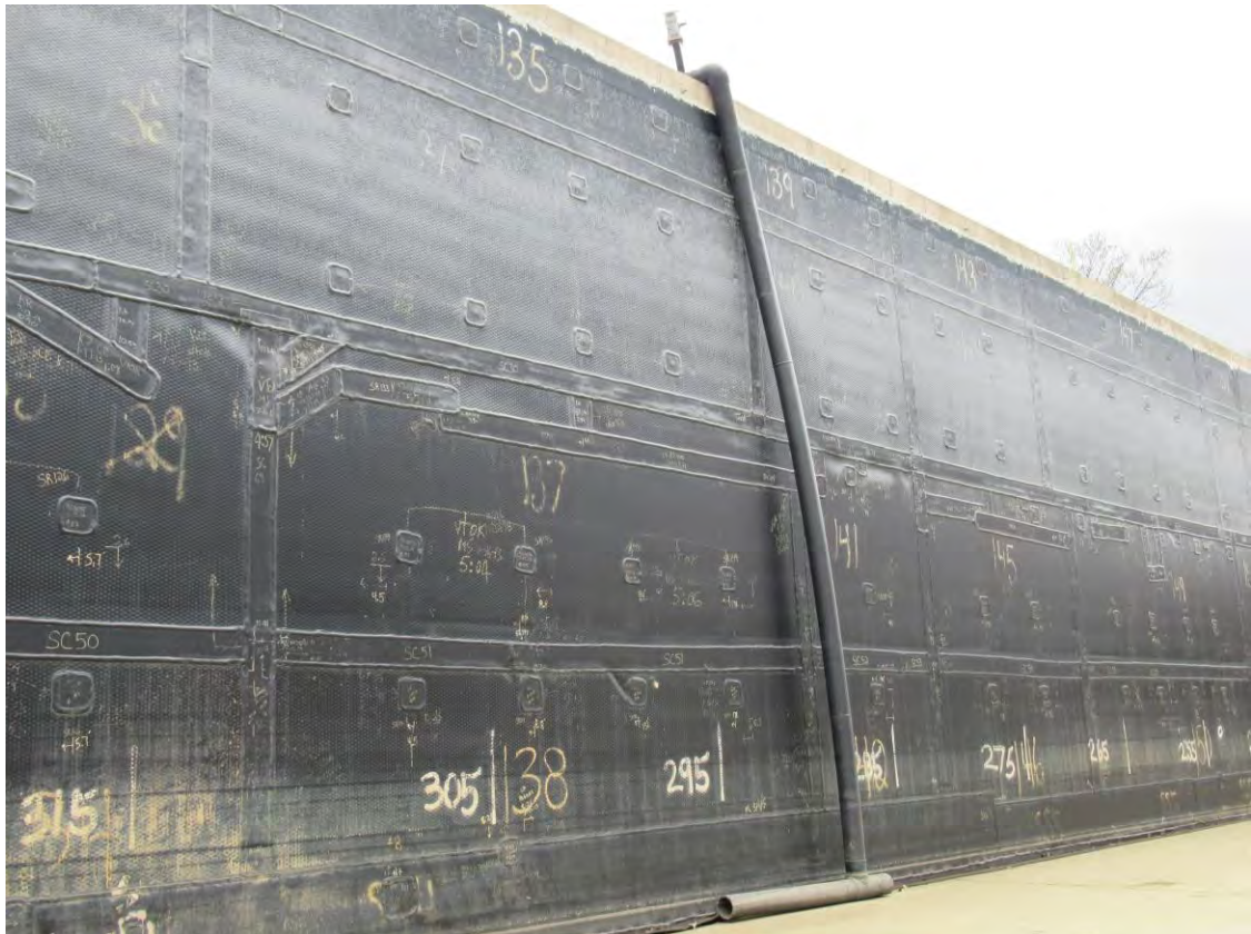
Temporary Fill Pipe for Hydrostatic Testing (Center of Southern Wall)
