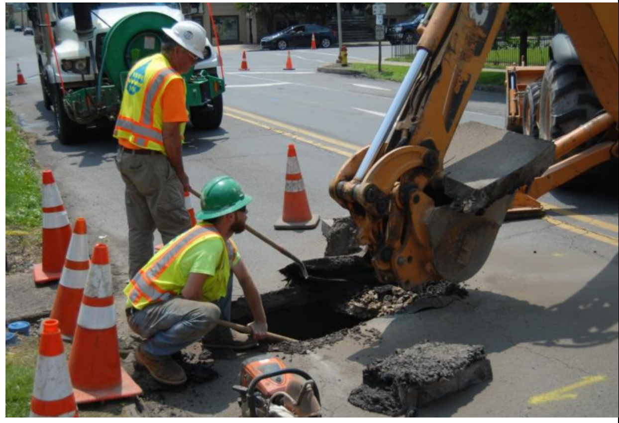
Figure 4.3.8-2 Large Sinkhole caused by sewer break in the City of Williamsport (Danneker, June 1, 2019).
