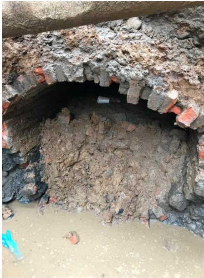
Figure 4.3.8-3 Large Sinkhole caused by sewer break in the City of Williamsport (Danneker, June 14, 2019).
