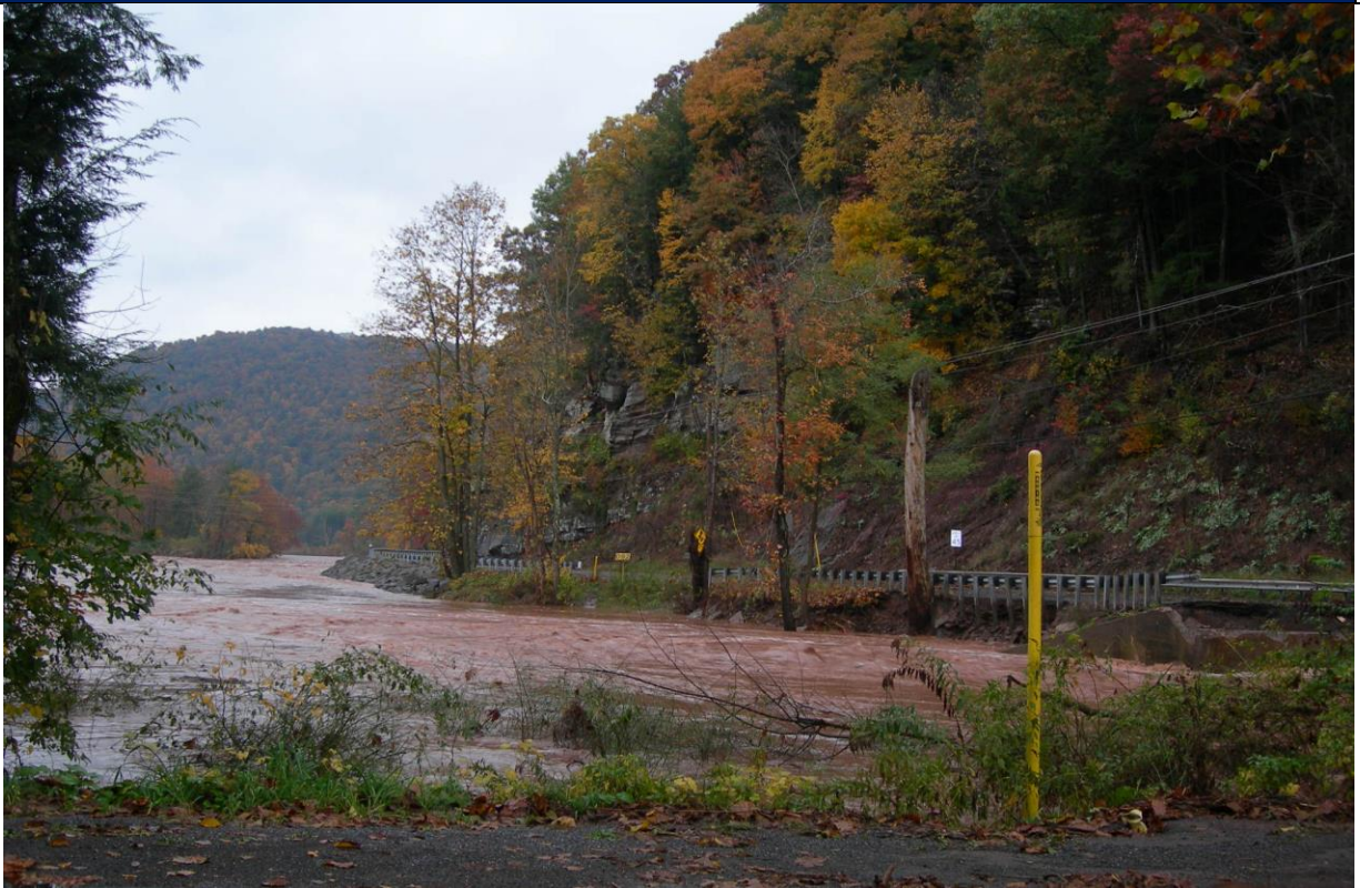
Figure 4.3.17-2 The yellow pipeline marker shows the location of the Sunoco pipeline rupture (Photograph courtesy of Carol Kafer / Loyalsock Watershed Association & Susan Phillips / StateImpact Pennsylvania).
