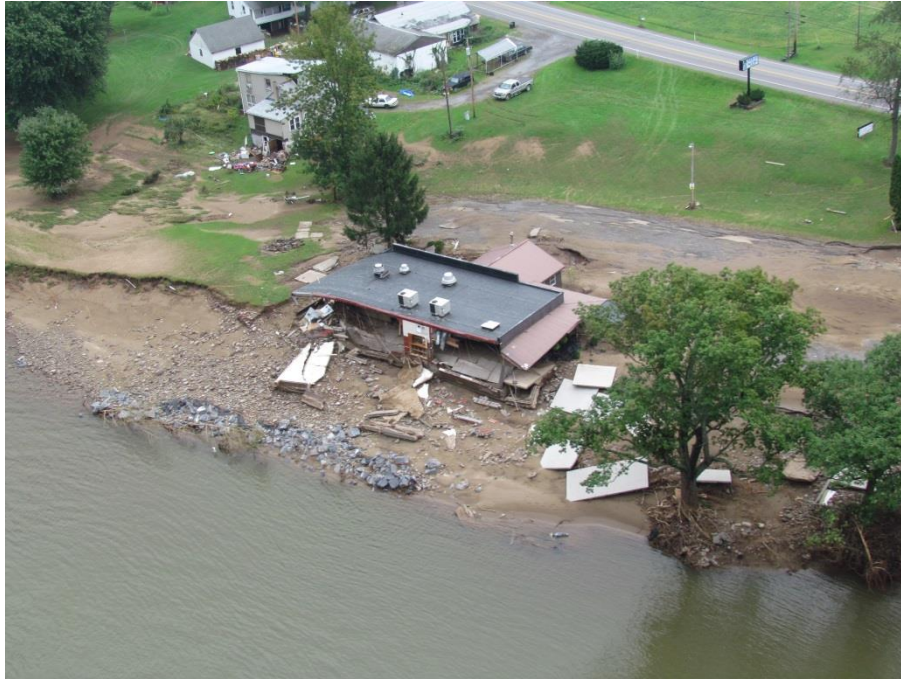
Figure 6.5-3 Pier 87 Bar and Grill before and after mitigation.
