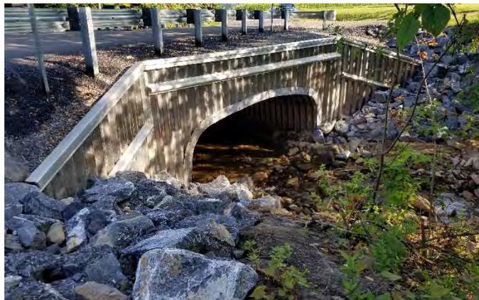
All four bridges in Bundle 1 were replaced with Aluminum Box Culverts, an innovative and cost-effective solution for municipalities to replace aging infrastructure. These structures also provide ample environmental benefits, namely the natural stream bottom which was used in all four of the bridges replaced in 2021 as part of the first bundle.
