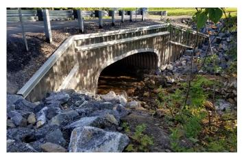
All four bridges in Bundle 1 were replaced with Aluminum Box Culverts, an innovative and cost-effective solution for municipalities to replace aging infrastructure. These structures also provide ample environmental benefits, namely the natural stream bottom which was used in all four of the bridges replaced in 2021 as part of the first bundle.
