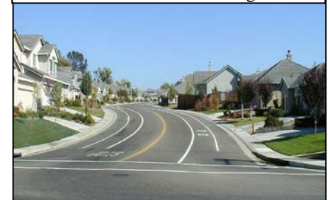
Example of Bike Lanes with On-Street Parking
