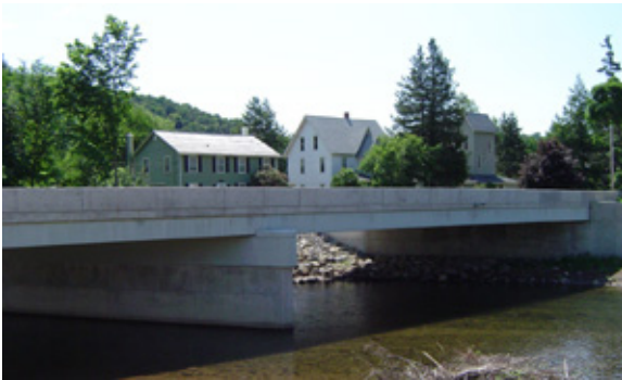
Recently replaced Muncy Creek Bridge in Picture Rocks
