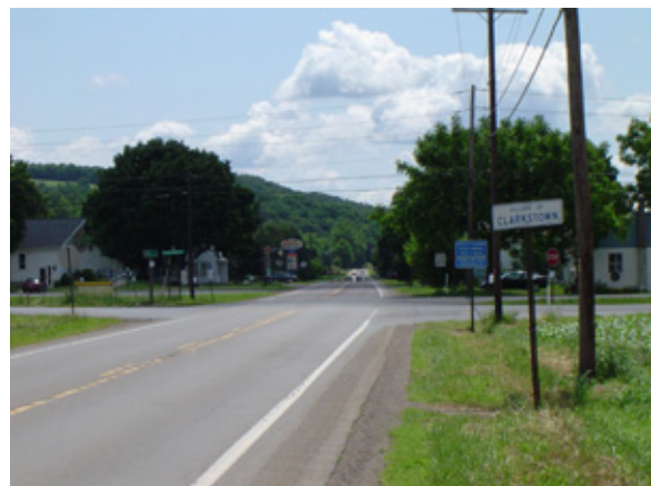
PA 442 looking east into Clarkstown
