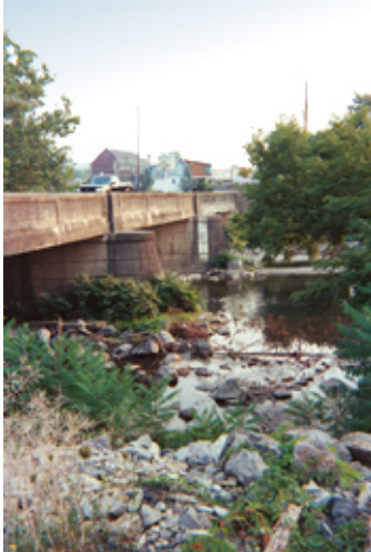
Muncy Creek Bridge
