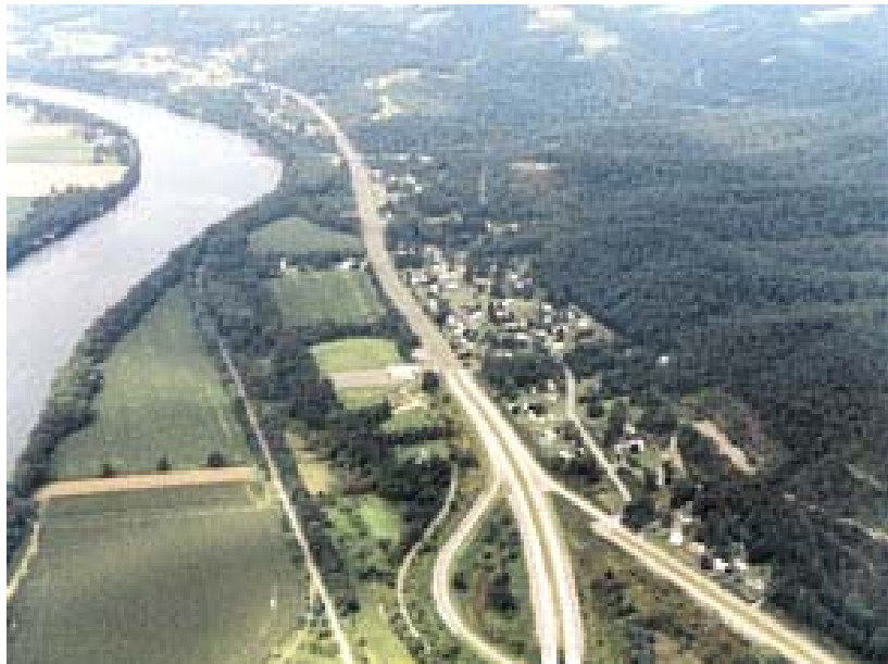
View of US 220/Future I-99 corridor in Woodward Township, where study of the land use impacts of the highway improvement has begun.
