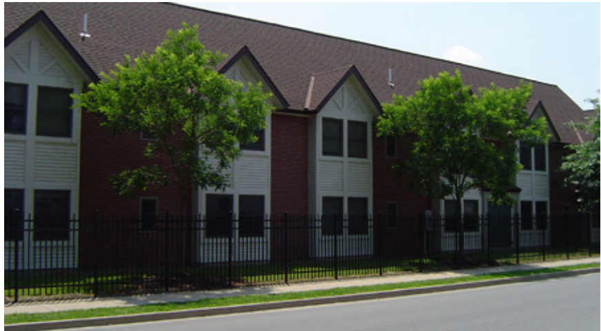
Apartment housing in Williamsport
