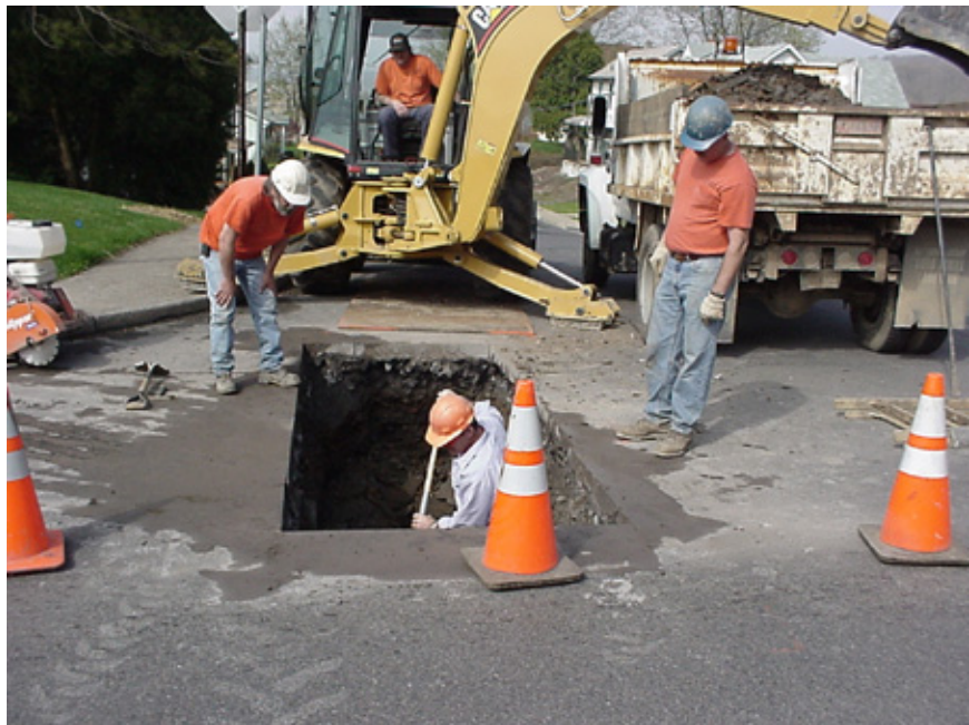
Infrastructure maintenance and repair in the Greater Williamsport Alliance Planning Area
