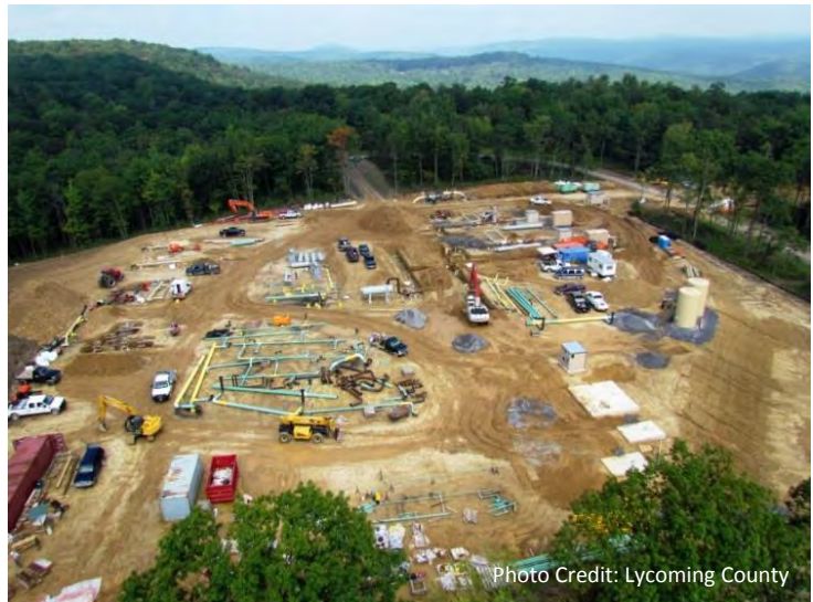
Ogontz East Compressor Station
