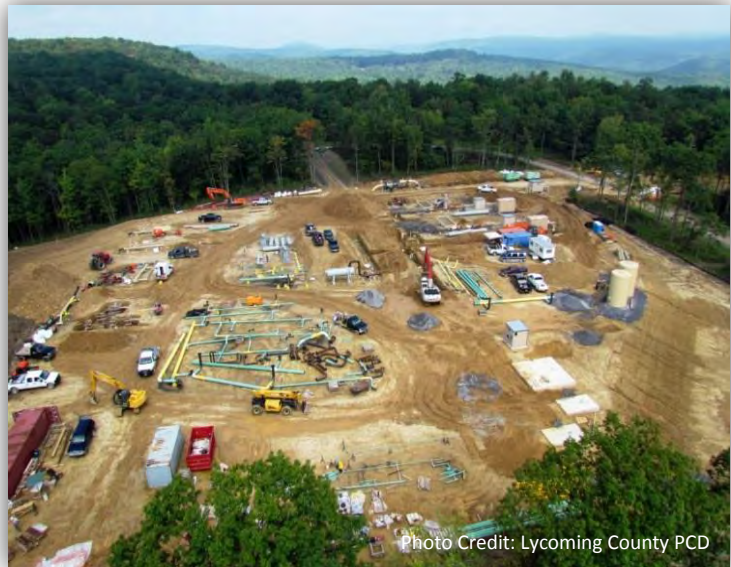
Ogontz East Compressor Station
