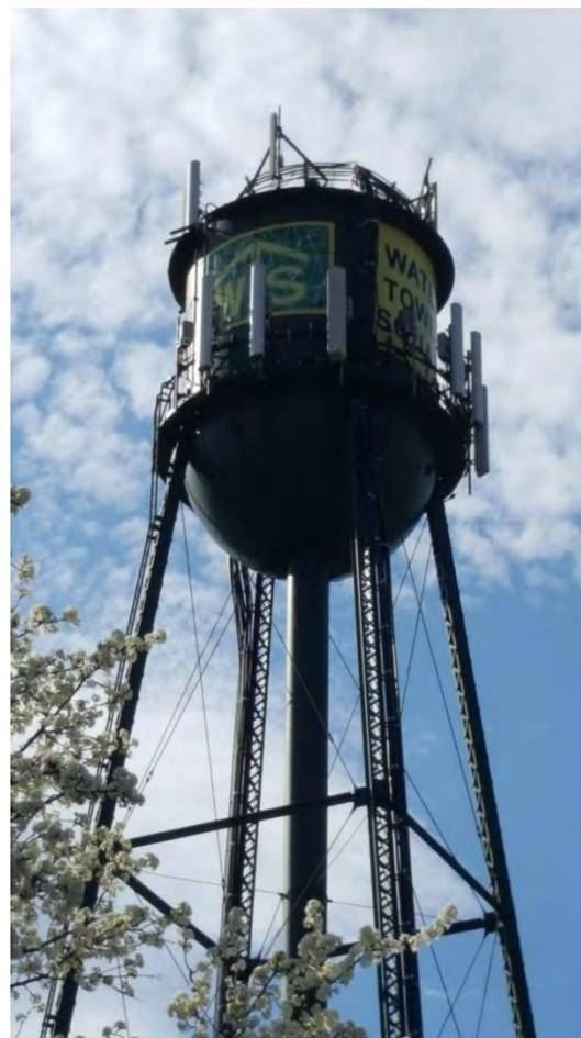
*Cellular antennae collocation utilizing existing vertical infrastructure has allowed cellular providers to provide coverage without building new towers in urban environments.*
