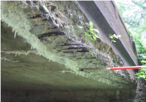
Severe spalling, cracking, and exposed, severely rusted rebar—T-506 over Daugherty's Run, Lewis Township
