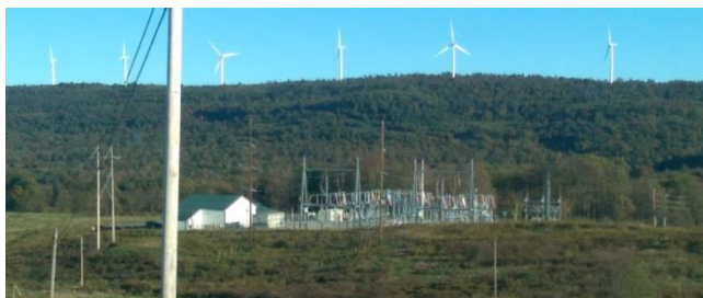
Laurel Hill Wind Energy Facility Substation with turbines on the ridge in the background
