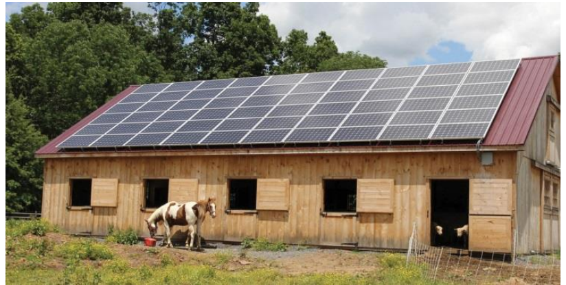
14.4 kW Agricultural Roof Mount, Kintnersville, PA Source: Paradise Energy Solutions, LLC
