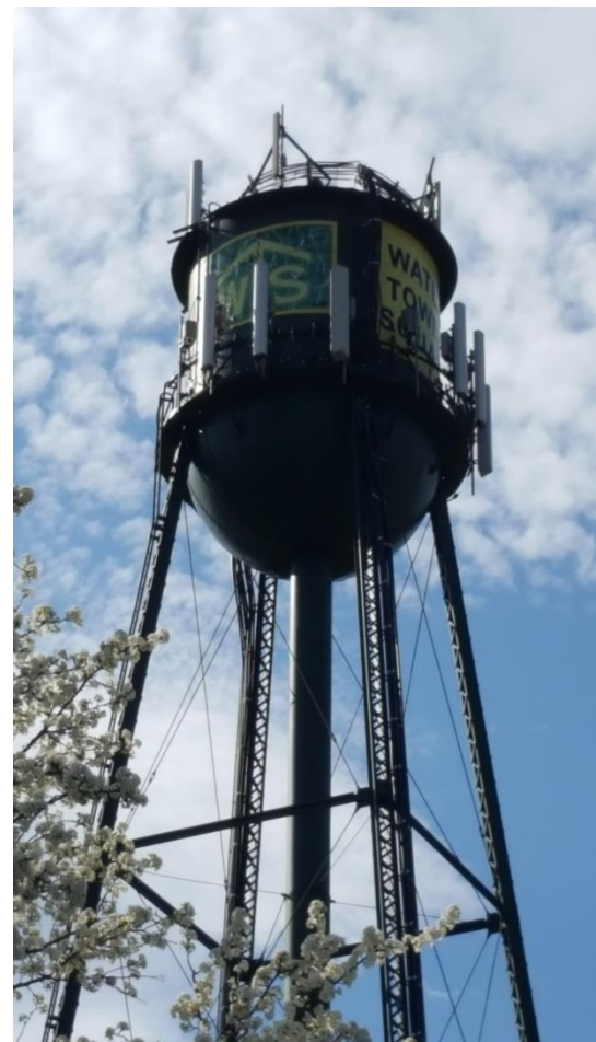
Cellular antennae collocation utilizing existing vertical infrastructure has allowed cellular providers to provide coverage without building new towers in urban environments. Source: PCD
