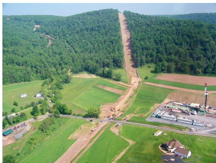
Natural gas pipeline under construction with a natural gas well pad Source: PCD
