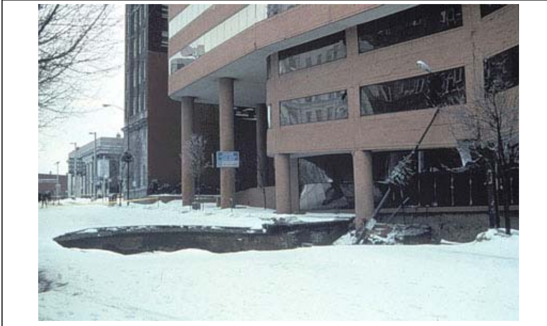
Figure 4.3.6-2 Sinkhole at Corporate Plaza Building in Allentown, Lehigh County, PA in February 1994 (Photography by William E. Kochanov – DCNR, 2009)
