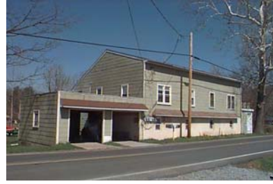
Street Address: 2995 Heshbon Rd. Parcel ID: 26-021-404 Lat/Long bldg dot: 41 17 10.45 N, -77 3 20.12 W FMV: $99,230
