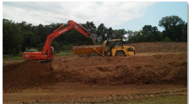
Photo 5: LCWSA's Wastewater Treatment Plant Improvements
