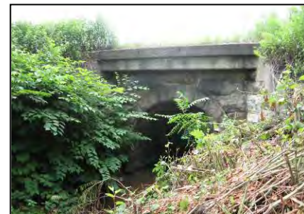
Existing Stone Arch Culvert over Quenshukeny Run
