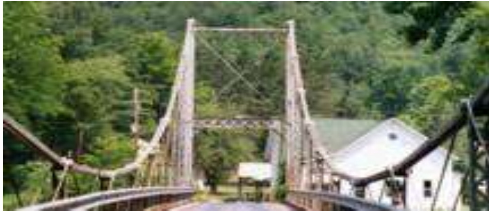
Historic English Center Suspension Bridge
