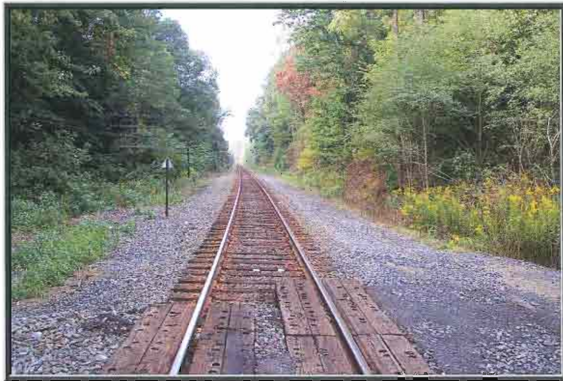
At-grade crossing of Norfolk Southern active rail line.
