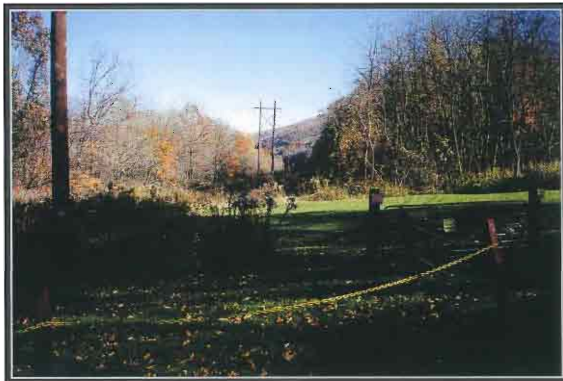
This is the access to the power line road directly off Sylvan Dell Road.
