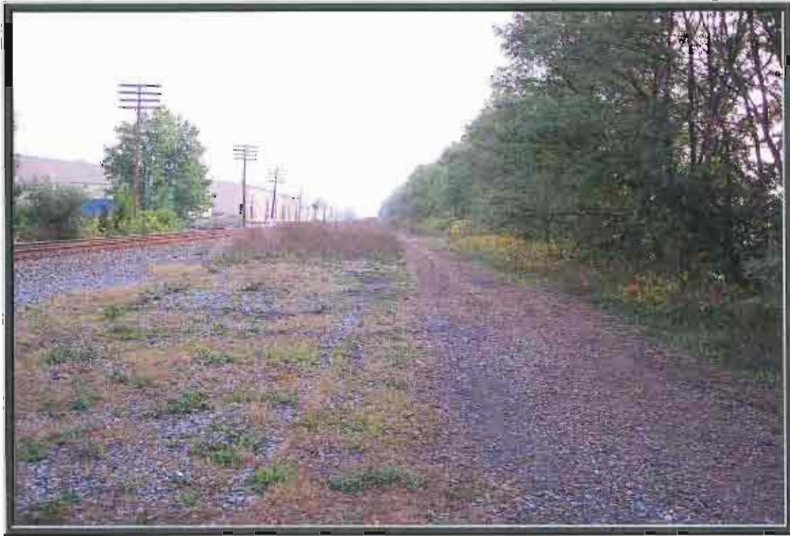
Norfolk Southern right-of-way near Montgomery.
