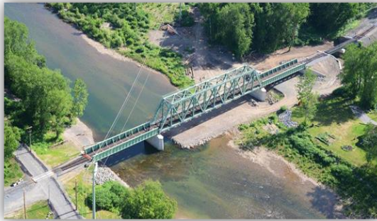
Loyalsock Creek Railroad Bridge
