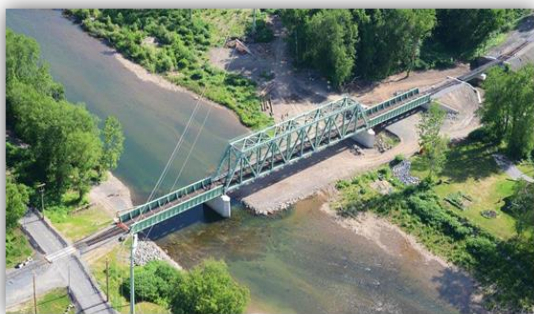
Loyalsock Creek Railroad Bridge
