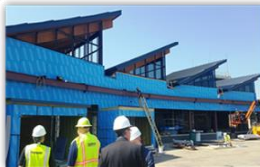
Williamsport Regional New Airport Terminal
