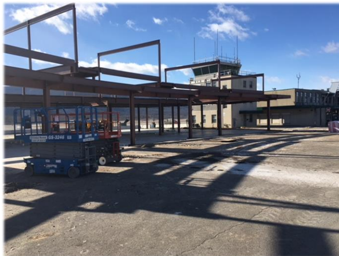
New Airport Terminal Construction, 2017
