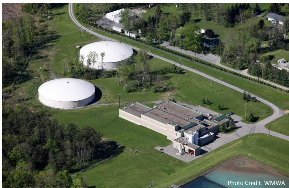
WMWA Water Filtration Plant in Armstrong Township
