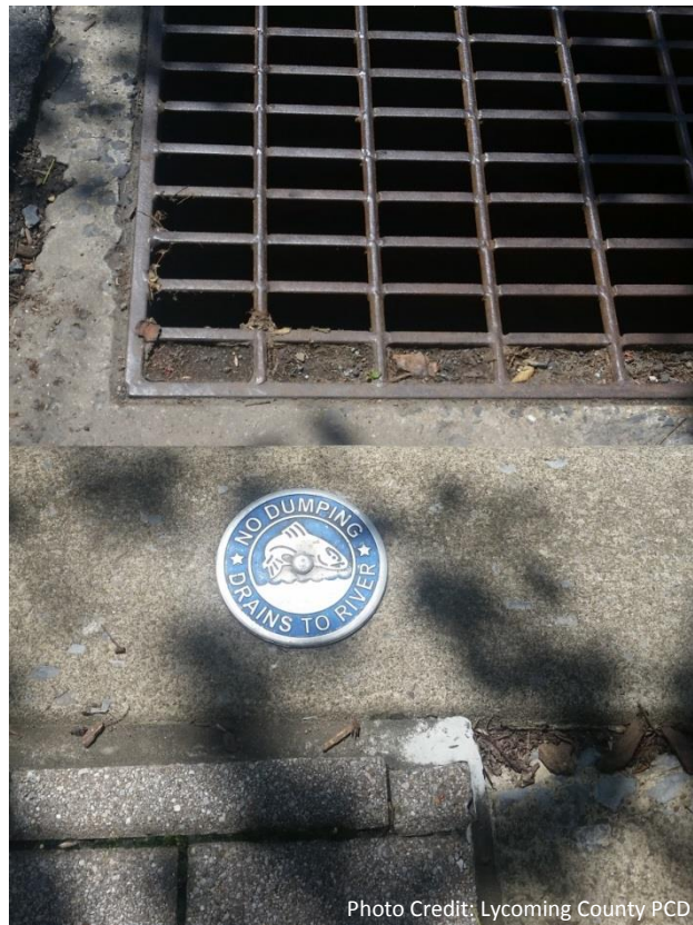
One of many “No Dumping” seals placed throughout the City as a way to promote proper water protection
