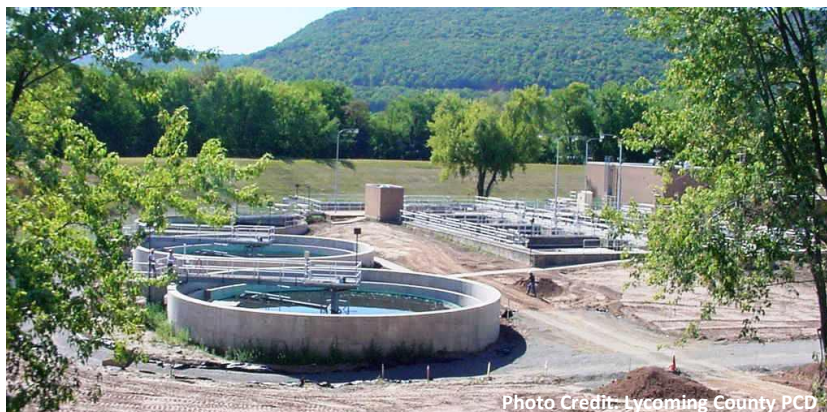
Photo Credit: Lycoming County PCD WSA West Treatment Plant Expansion
