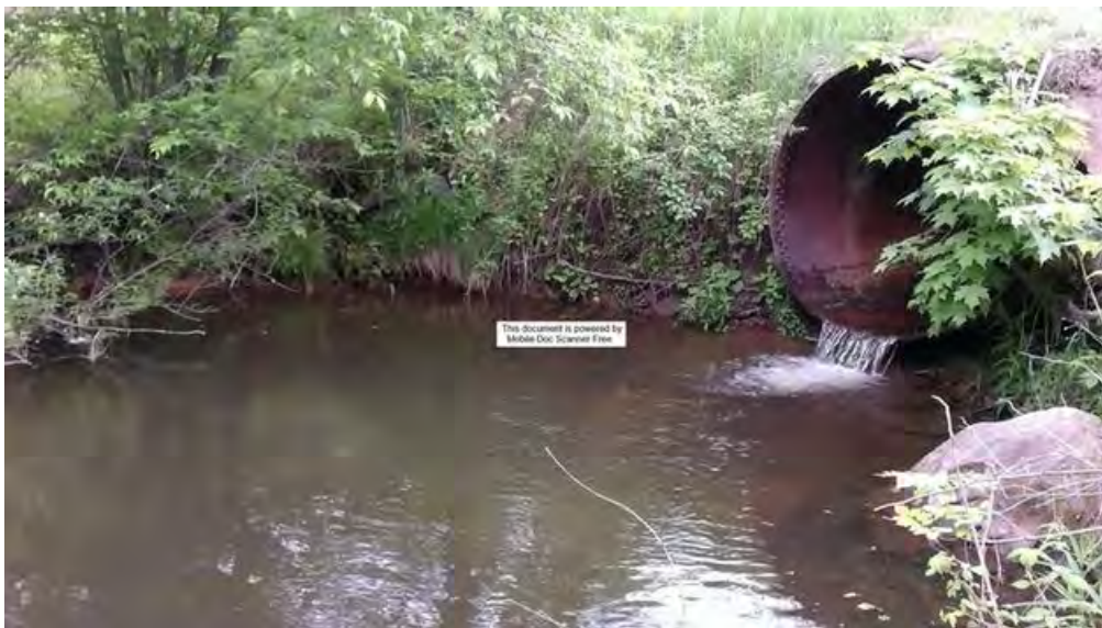
Figure 22. Culvert on Hawk Run (outlet)
