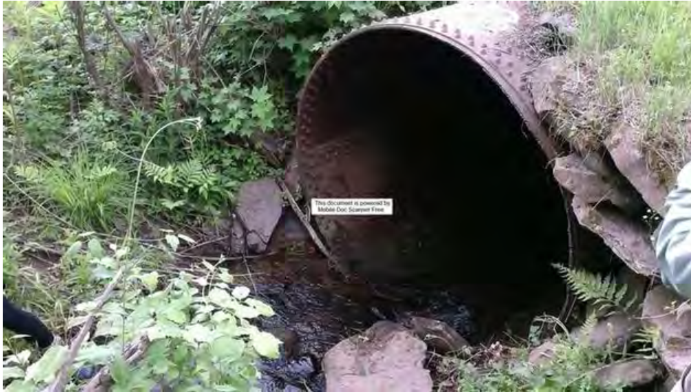
Figure 21. Culvert on Hawk Run (inlet)
