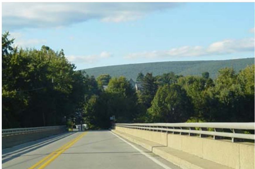
Route 54 river bridge into Montgomery Borough
