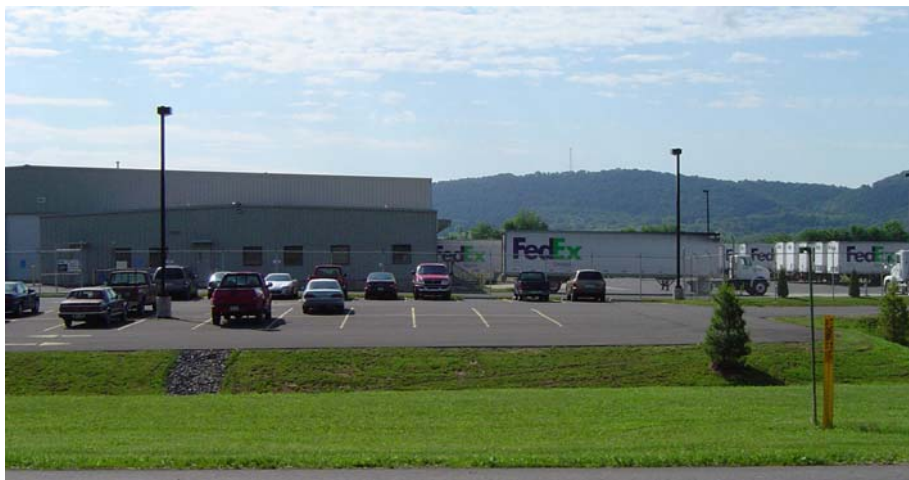
FedEx site development in Clinton Township
