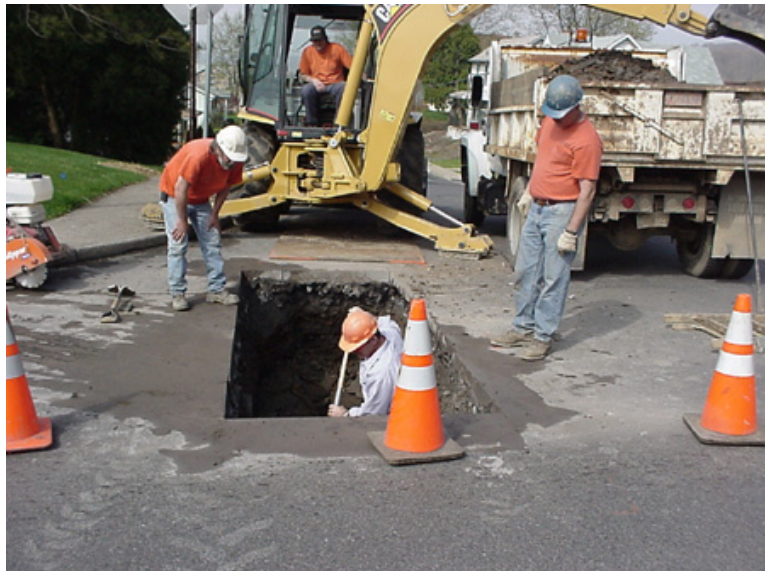
Maintenance crew in the Williamsport area
