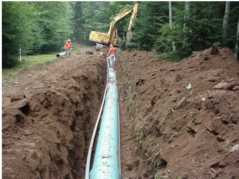
Pipe installation along US 220
