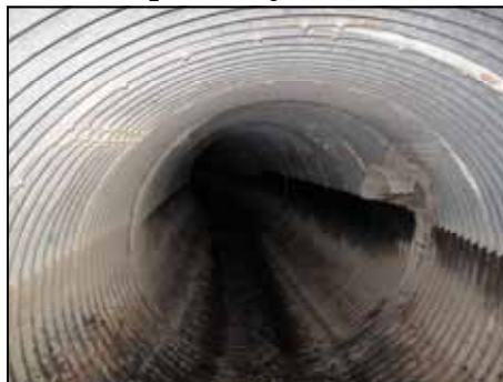
Deteriorating Culvert
