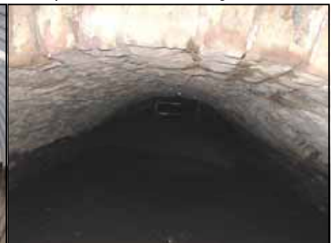
Failing Stone Arch Enclosure
