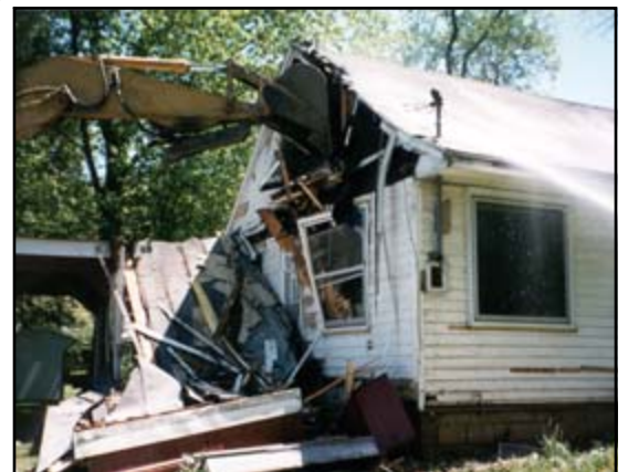
Demolition of flood-damaged home along Lycoming Creek
