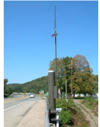
Hepburnville ultrasonic stream level gage
