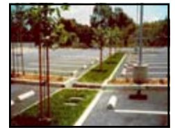
Examples of stormwater BMPs (Best Management Practices) include (clockwise from top left): Bioswales; rain gardens; pervious pavements; curb breaks; and parking lot infiltration areas. Stormwater is filtered and re-charges groundwater supplies, rather than running off into streams during wet weather events. DEP is currently performing studies to develop protocols for the calculation of nutrient credits for such BMPs.
