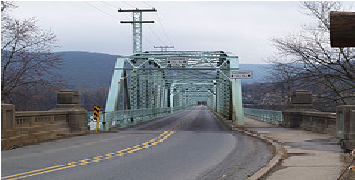
Existing Arch Street Bridge built in 1923
