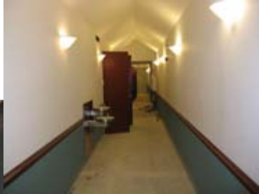
HOPE Enterprise Under Construction
