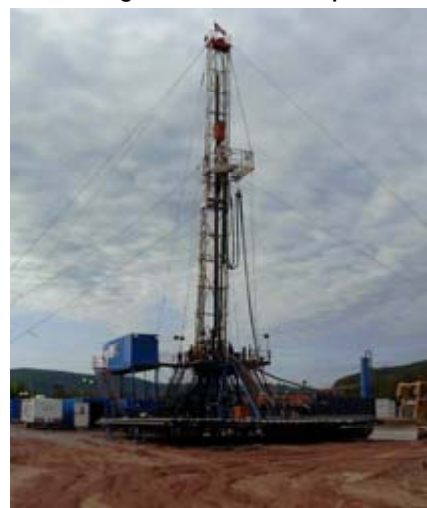
Drill rig at Penn Township site
