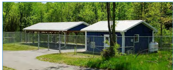
Brady Township's Small Treatment Plant Source: Staff photo
