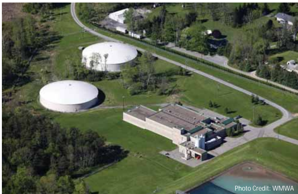
WMWA Water Filtration Plant in Armstrong Township
