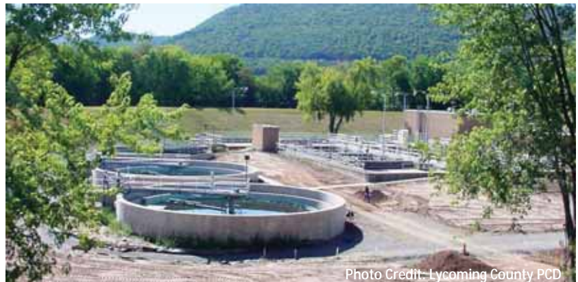
WSA West Treatment Plant Expansion
