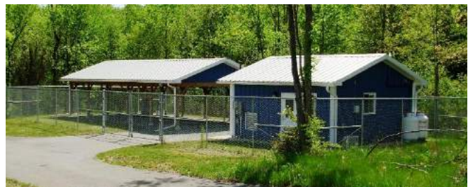
Brady Township's Small Treatment Plant
