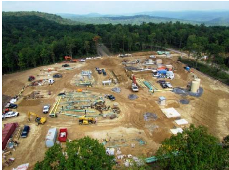
Ogontz East Compressor Station
