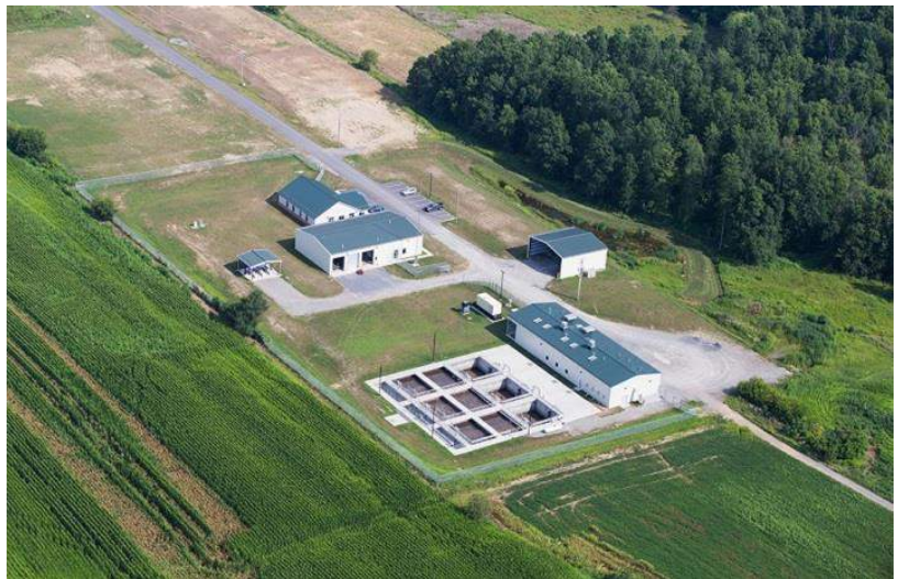
TVMA Wastewater Treatment Site
