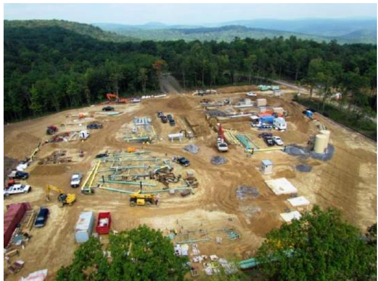
Ogontz East Compressor Station
