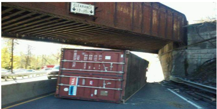
I-99 / US 220 PAT Structurally Deficient Bridges
