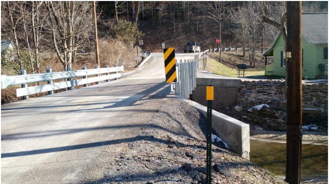
Woodward Township T369 Bridge Replacement
