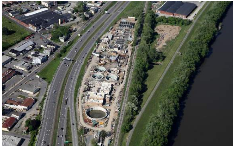
WSA Central Treatment Plant Expansion
