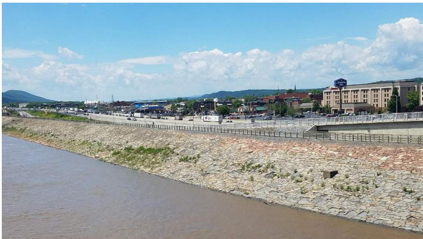
A view from the Susquehanna Riverwalk showing the Williamsport Levee protecting its downtown infrastructure
