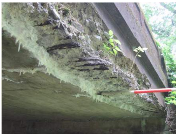
Structurally deficient bridge segment
