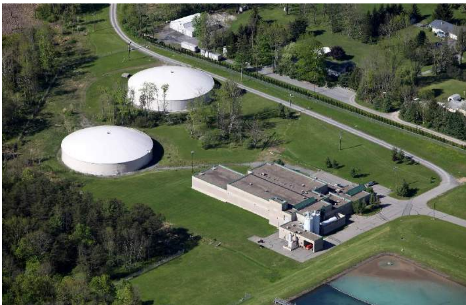
WMWA Water Filtration Plant in Armstrong Township
