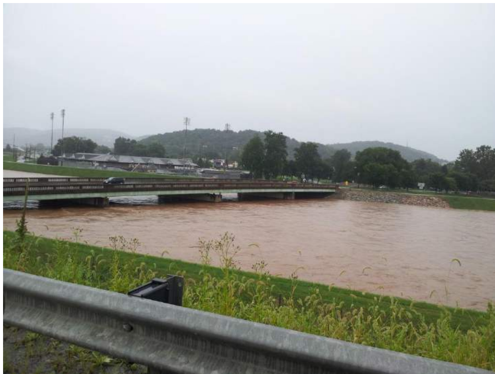
Planning area levee protecting nearby homes as flood levels rise during 2011’s Tropical Storm Lee
