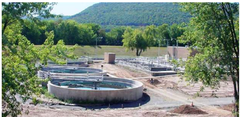
WSA West Treatment Plant Expansion
