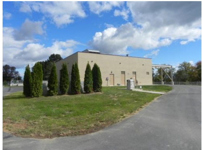
WBRA's new WWTP that serves four municipalities: Muncy and Montgomery Boroughs and Muncy Creek and Clinton Townships.
