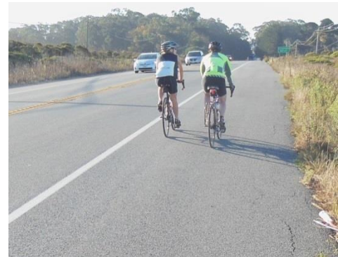
Wide shoulders allow cyclists to travel outside of the main travel lane. Source: thirdwavecyclingblog
