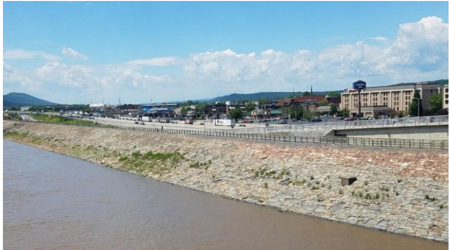
A view from the Susquehanna Riverwalk showing the Williamsport Levee protecting downtown infrastructure
