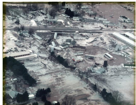
Flooding aftermath along Lycoming Creek Road in January 1996 Source: PCD
