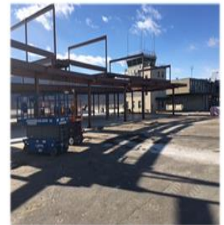
New Airport Terminal Construction, 2017
