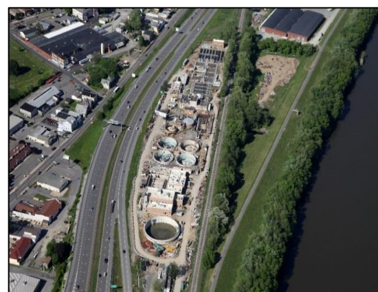
WSA's Central Wastewater Treatment Plant was a multi-million dollar expansion and technological upgrade to satisfy federal environmental regulations
