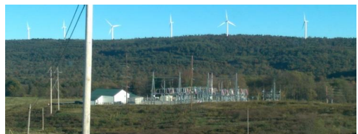
Laurel Hill Wind Energy Facility Substation with turbines on the ridge in the background
