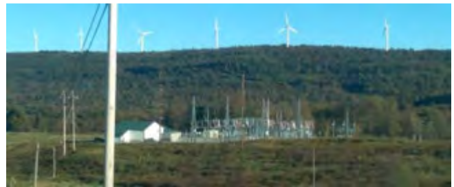
Laurel Hill Wind Energy Facility Substation with turbines on the ridge in the background
