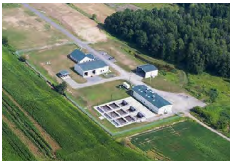
TVMA's new WWTP to serve Jersey Shore and urbanized areas of Porter and Nipponese Townships
