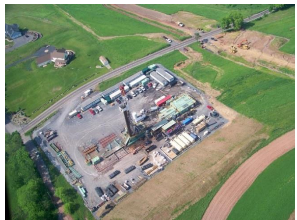
Natural Gas Well Pad, Cogan House Township Source: PCD
