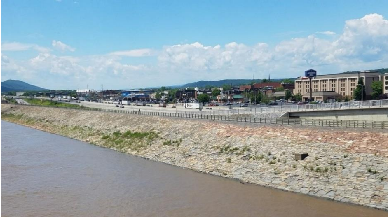
A view from the Susquehanna River Walk showing the Williamsport Levee protecting downtown infrastructure Source: PCD
