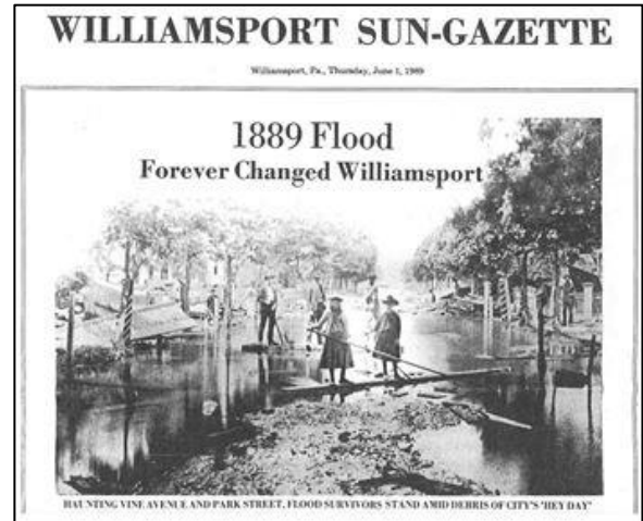
Newspaper article depicting children using a raft from debris following the 1889 flood Source: Williamsport Sun Gazette
