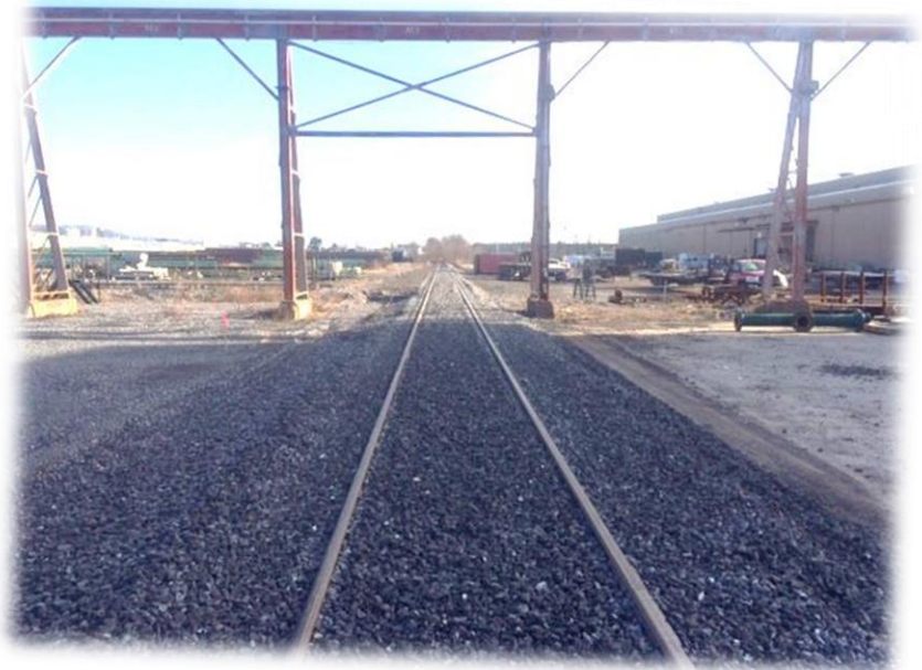
Freight rail siding with Overhead Crane, Reach Rd. Industrial Park Area, Williamsport Source: PCD
