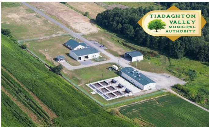
TVMA Sanitary Sewer Plant completed 2014 Source: Larson Design Group
