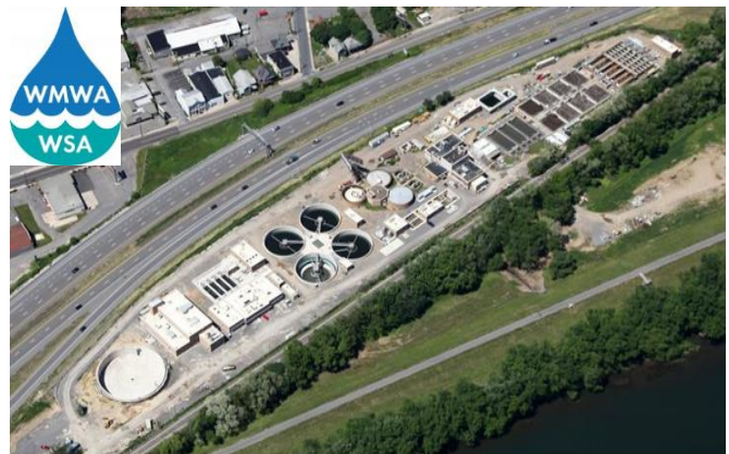
WMWA-WSA Central Plant upgrades completed 2013 Source: WMWA-WSA
