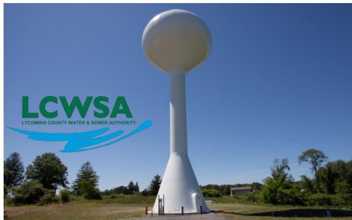
LCWSA's recently constructed water tower Source: hrg-inc.com
