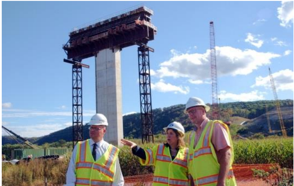
PennDOT Secretary Leslie Richards Tours CSV T Project Site, 10/2017 Source: PennLive.com
