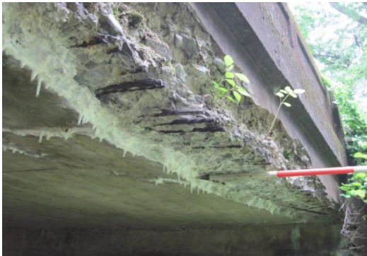
Severe spalling, cracking, and exposed, severely rusted rebar—T-506 over Daugherty's Run, Lewis Township Source: Larson Design Group
