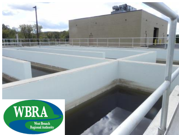
WBRA Sanitary Sewer Plant constructed 2015 Source: PCD
