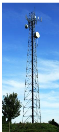
Microwave Communication Tower Source: PCD
