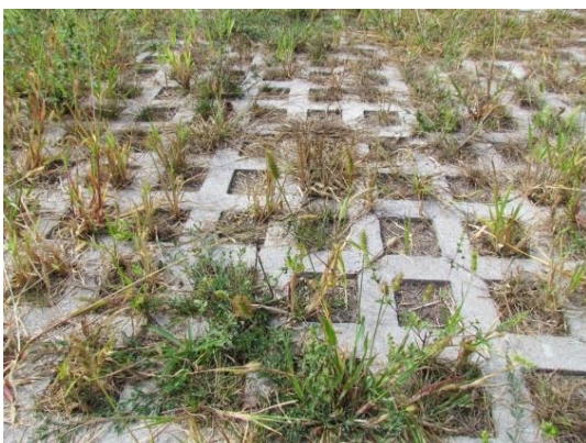
Pervious pavement at the Jersey Shore Public Library Source: PCD
