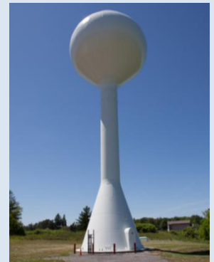
LCWSA’s new water storage tank in Grey Fox Plaza, Fairfield Township Source: PCD
