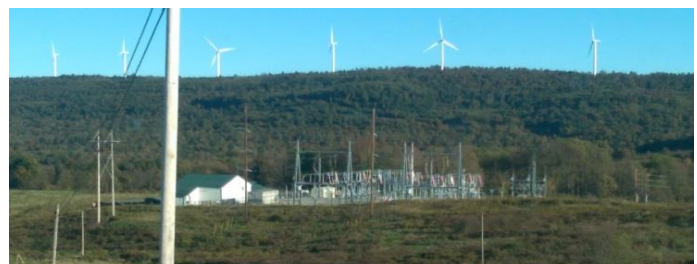
Laurel Hill Wind Energy Facility Substation with turbines on the ridge in the background Source: PCD
