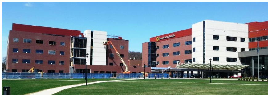
The Health Innovation Center during construction (left) with the completed Patient Tower (right) at Williamsport Regional Medical Center
