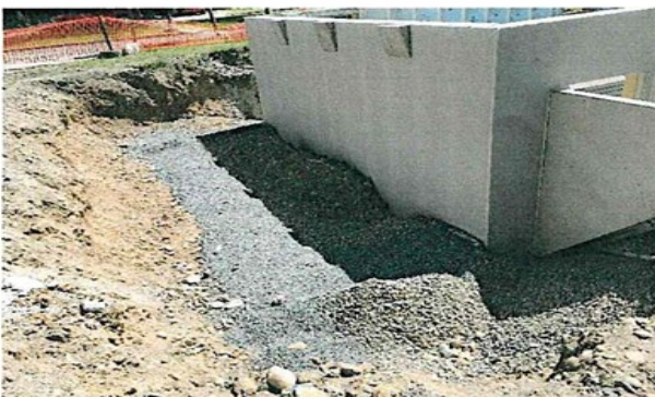
June 14. Wall backfill.
