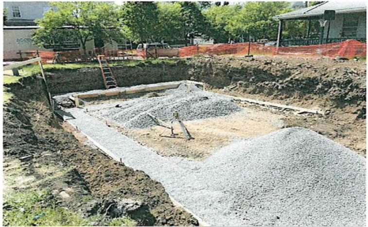
May 23. Forming stone for foundation walls.
