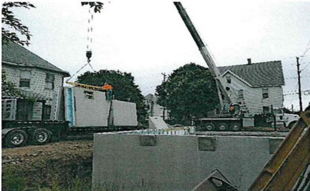
June 2. Crane setting walls.
