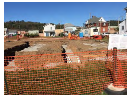
Site preparation work for the double home in the BNIP neighborhood
