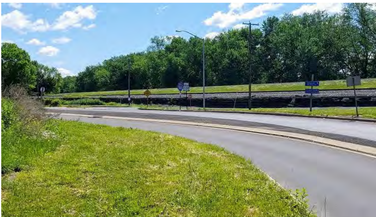
View of Phase 2 location where the pedestrian ramp and at grade crossing with the Lycoming Valley Railroad will be installed
