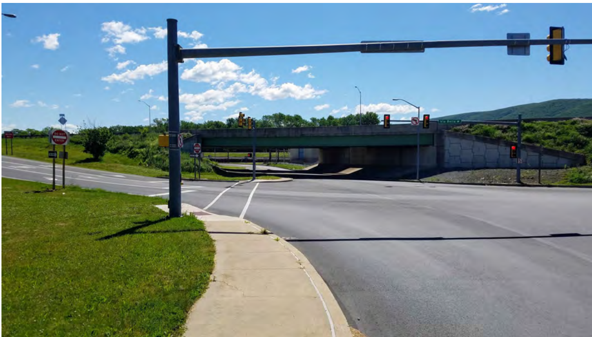
View of trail connector alignment facing South from intersection of Via Bella and Basin Street
