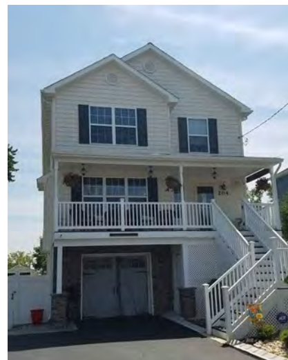
An elevated home post Hurricane Sandy in Iselin, NJ
