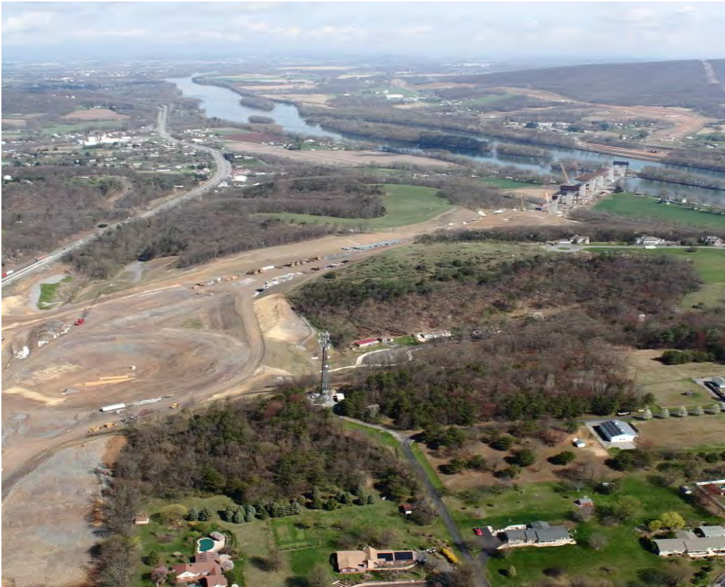
Looking North from County Line Road at work between US 15 and River
