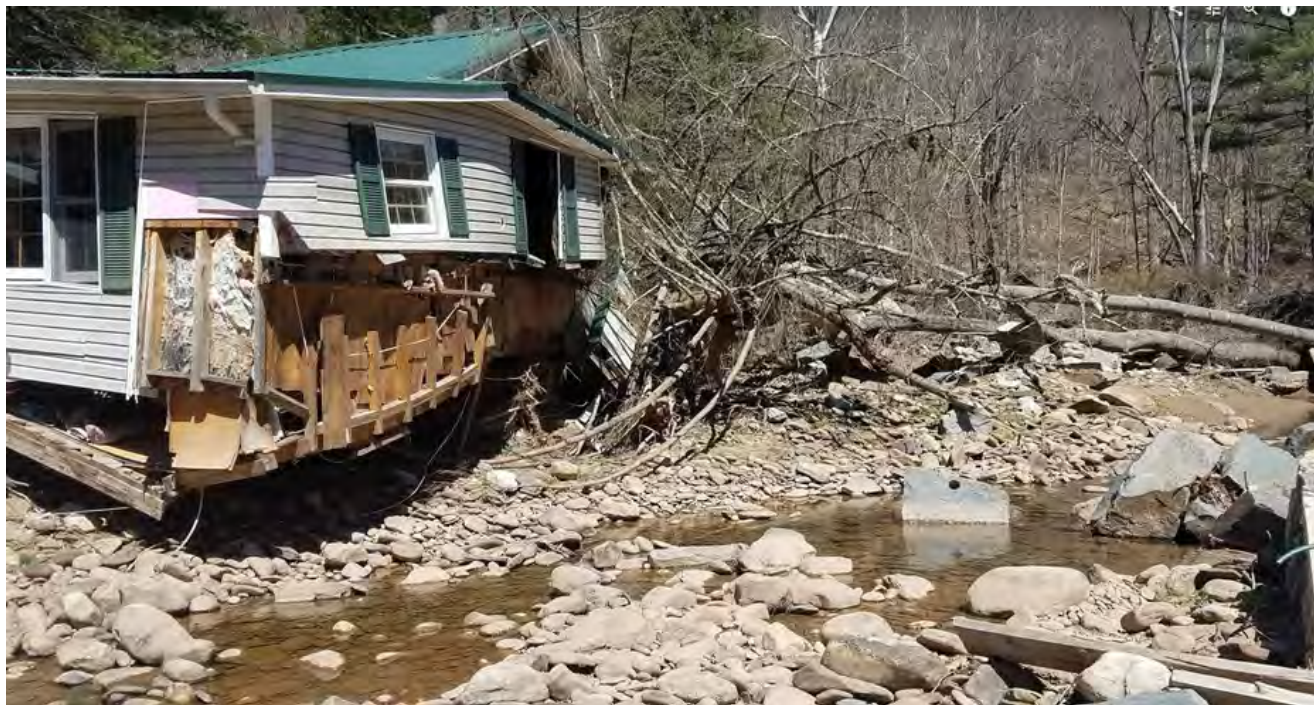
An example of a home damaged during a flooding event in McIntyre Township. The County subsequently applied for a Hazard Mitigation Buyout Grant through FEMA in 2017.
