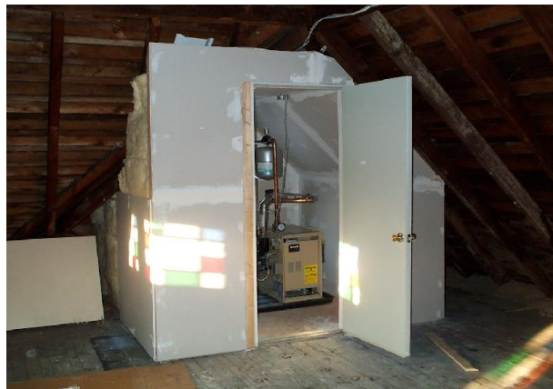
Heating plant placed in attic above possible floodwaters
